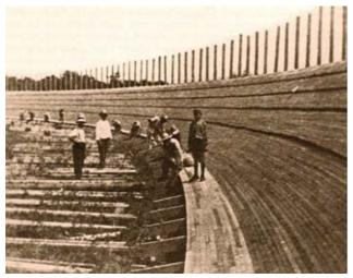
constructors, hoping for higher speeds, increased the angle of banking to 40 and even 50 degrees. Not until a decade after the building of the Playa del Ray, did board track builders begin to make use of knowledge the railway companies had held for years and employ the principle of the Spiral Easement Curve.
